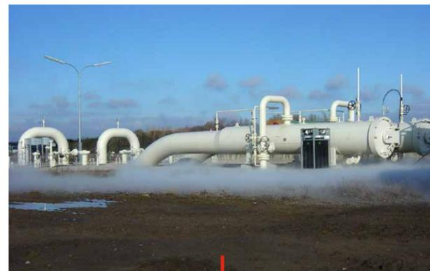
Pig Trap with HEAT Quick Opening Closure
