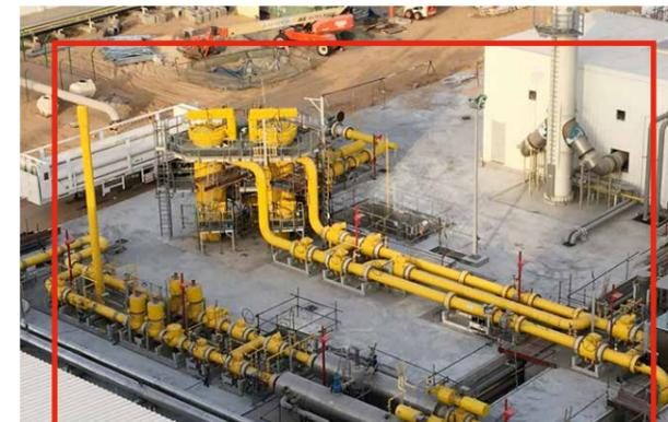
Hamriyah (UAE) power plant Fuel gas supply system with hot water heating, 205 m<sup>3</sup> buffer and Switch over buffer conditioning system
