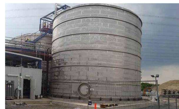
Aqueous ammonia storage tanks 2x 1.100 m<sup>3</sup> double walled (WHG) - site manufacturing
