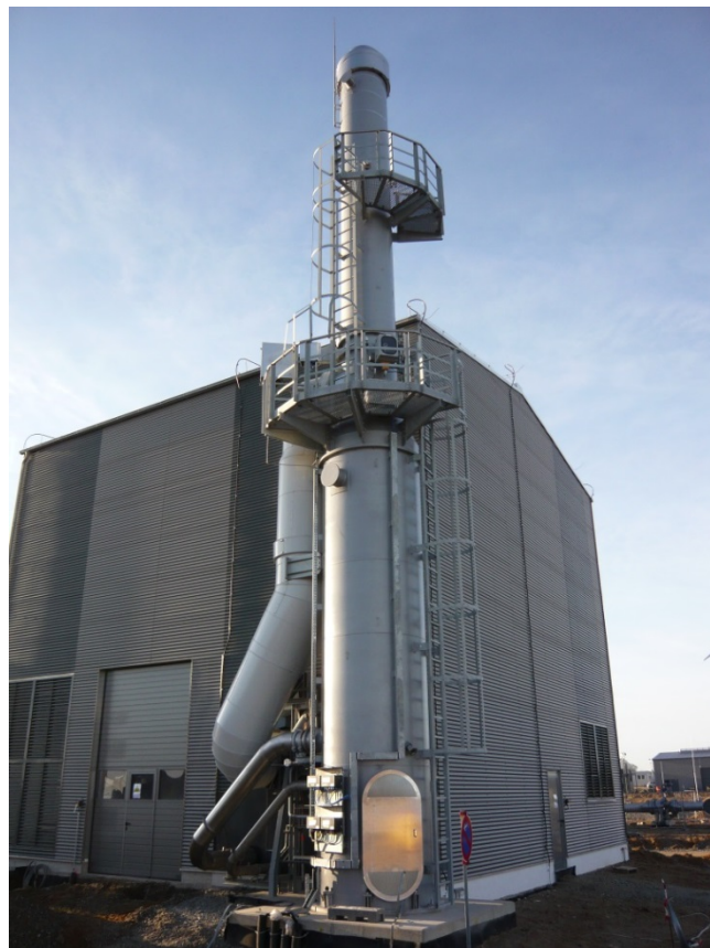
Reboiler for 6.500 kg TEG/h and horizontal incinerator 900 kW
