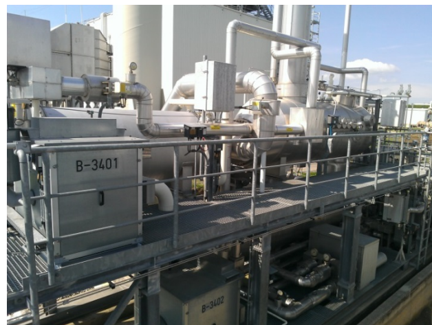
Reboiler for 6.500 kg TEG/h and horizontal incinerator 900 kW
