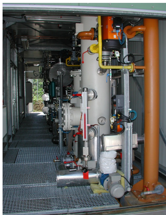
Condensate separator with drain pump
