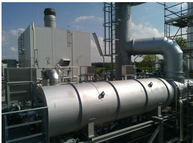
Reboiler for 6.500 kg TEG/h and horizontal incinerator 900 kW
