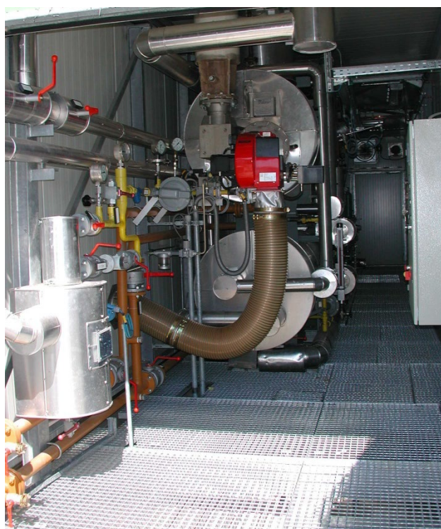
Reboiler 350 kW with burner and surge drum
